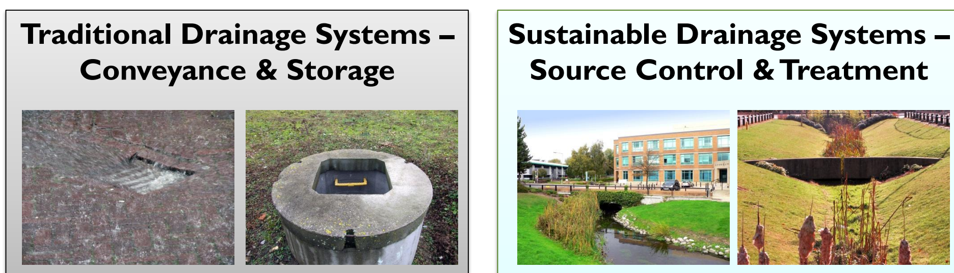
Figure 1 – examples of both conventional and sustainable drainage systems (images courtesy of Micro Drainage).
