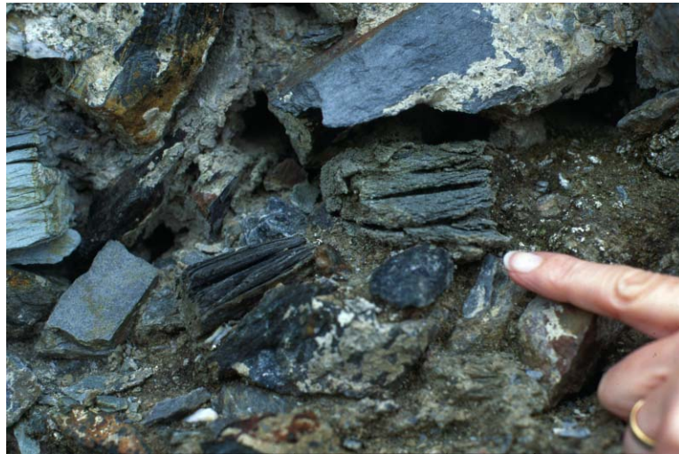
Figure 2-11. Strongly exfoliated mudstone aggregate in mass concrete. Ruined mill building at West Wheal Kitty Mine, near St Agnes.
