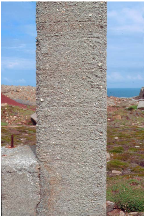
Figure 2-17. Mass concrete pillar at Levant Mine, near St Just in Penwith.
